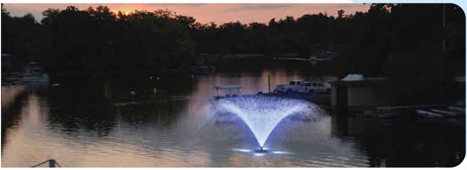
Safe-Rains floating fountains Control Panel/
